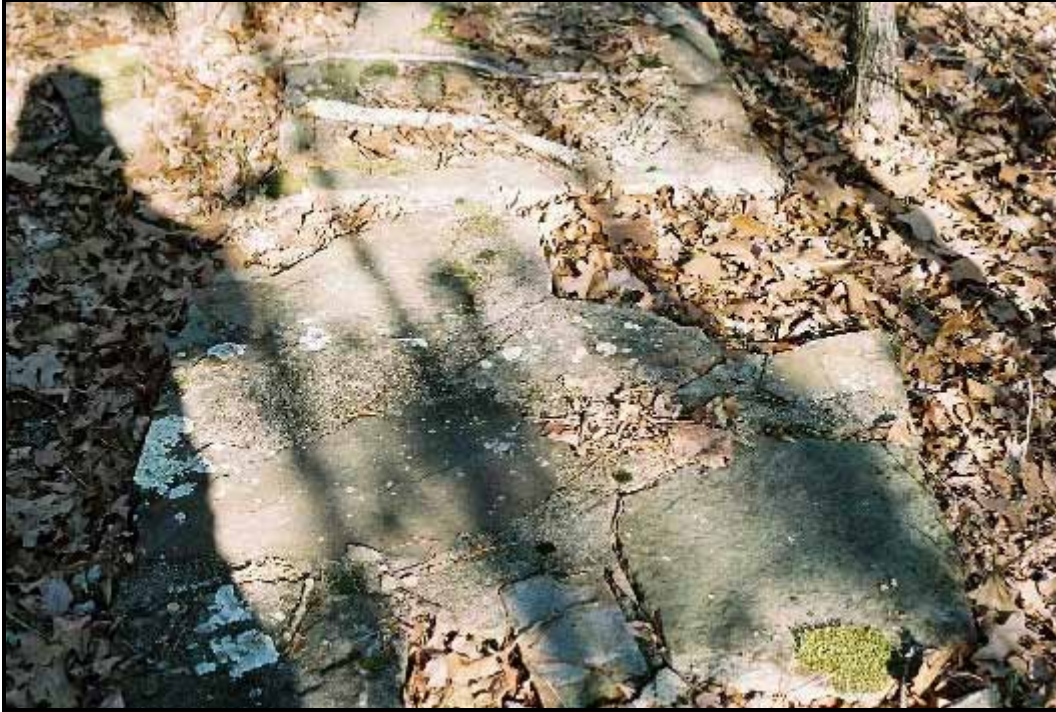
Contributing Structural Element E (1940-41 Stone Sidewalk)
