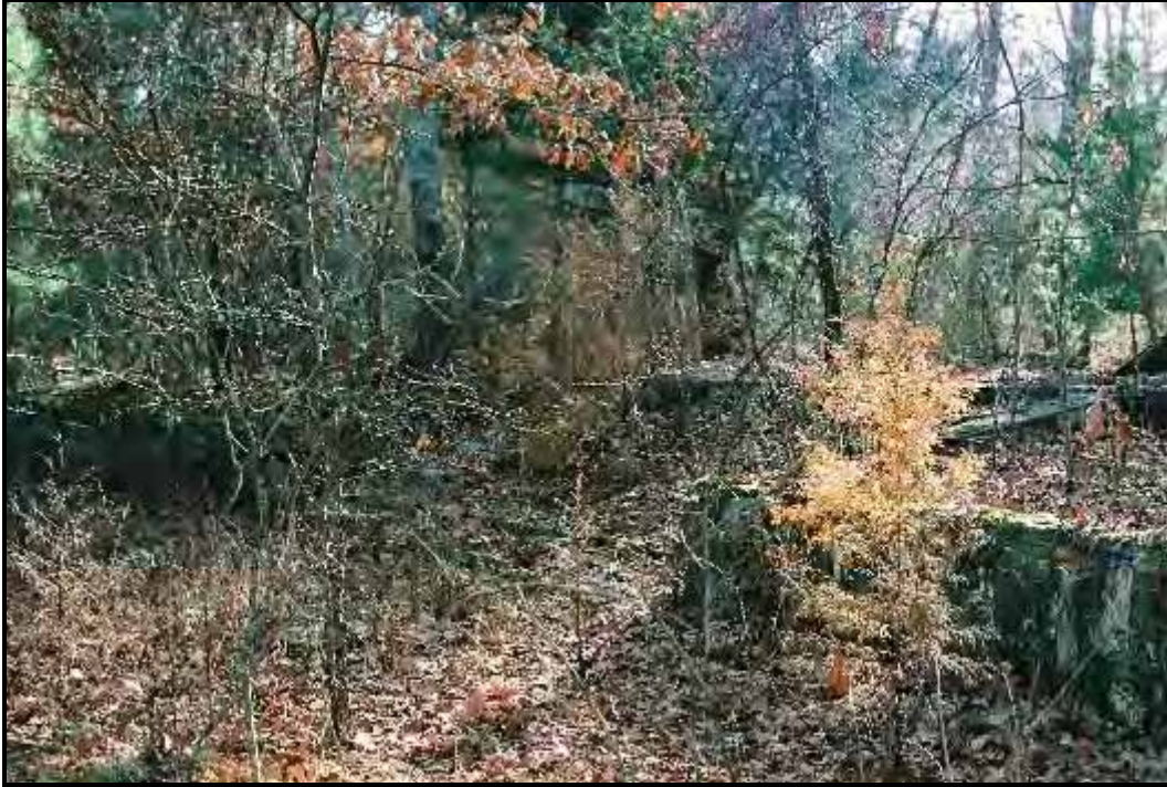
Contributing Structural Element A (1943 Stone Culvert and Stone Steps/semi-circular Retaining Wall)
