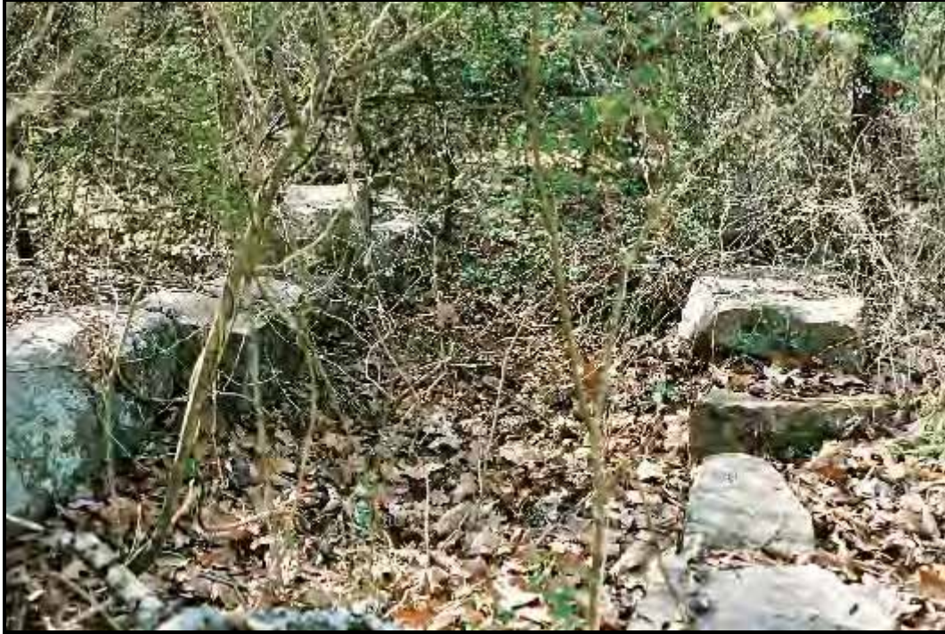
Contributing Structural Element D (1940-41 Stone Retaining Wall/Steps)
