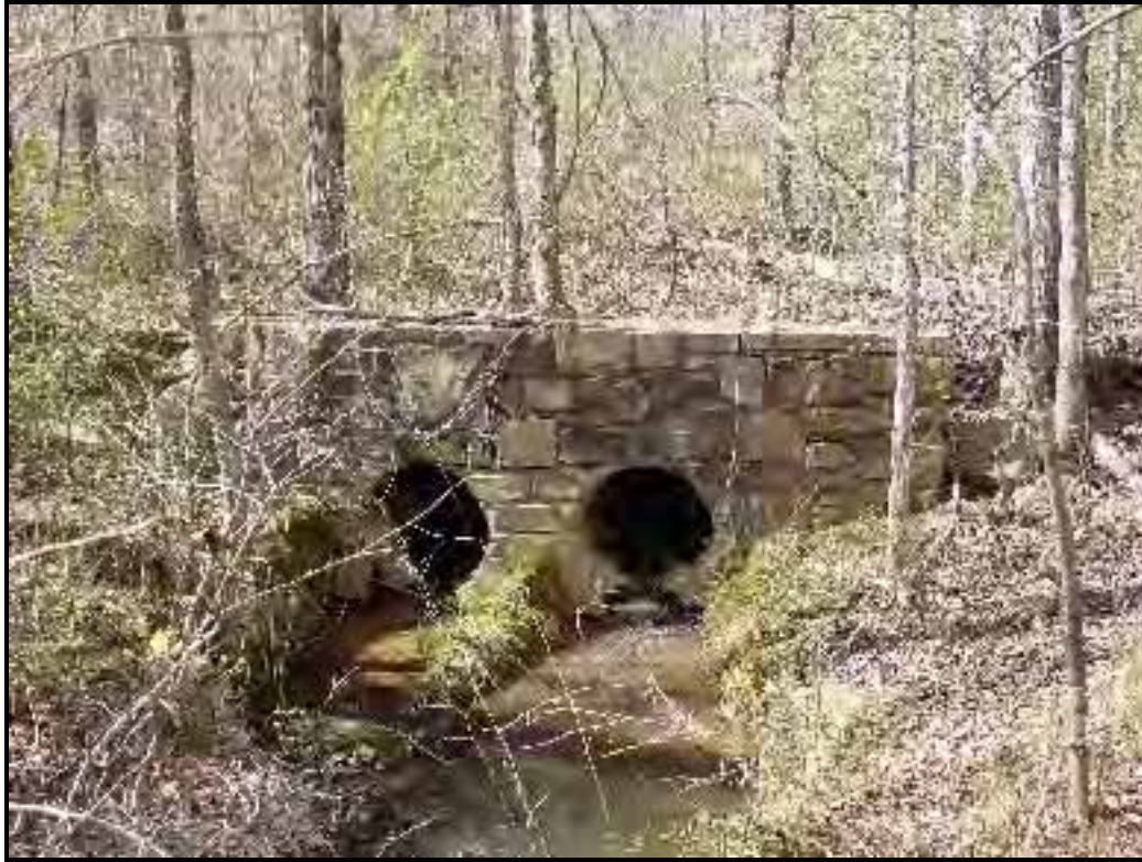
Camp Robinson Bridge #2 (1943 Stone Culvert)
